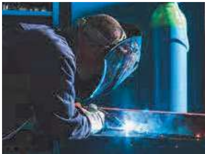
Manual MAG welding
